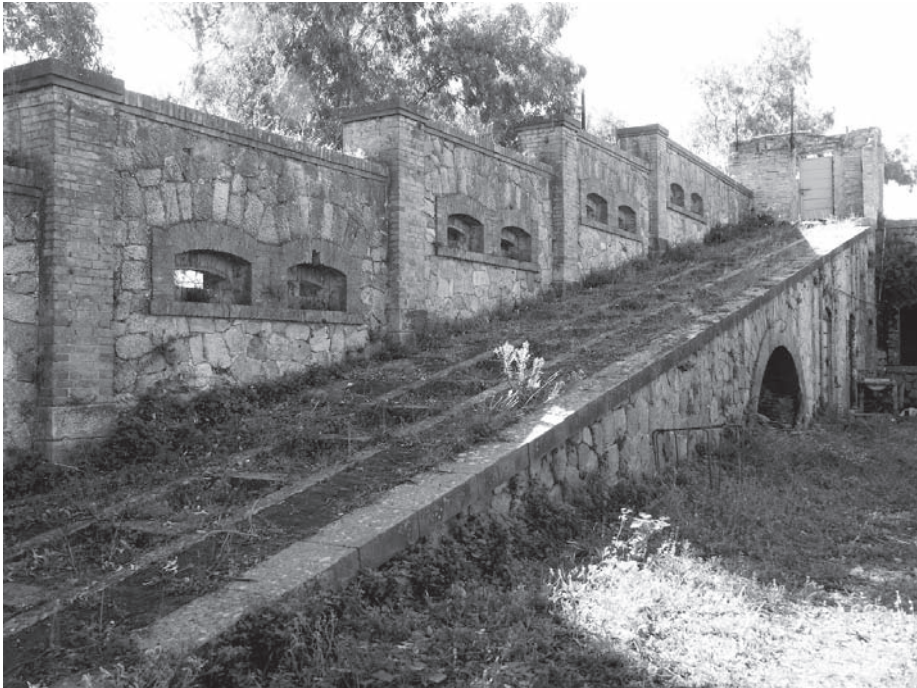
Fig. 12. Coast Battery Monte dei Centri 12S, detail of the ramp to the howitzers.
