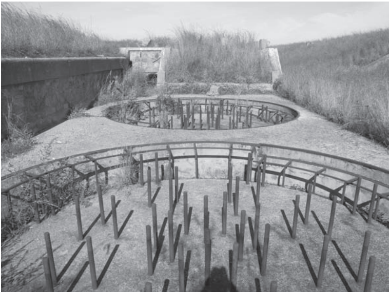
Fig. 8. Coast Battery Cimitero di Catona 5C, hooks of turntables Platforms for howitzers.
